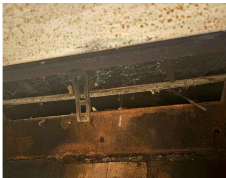
General - Interior: Chimney Location
